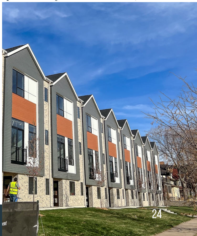
Figure 13: Middle housing under construction in Merriam Park, Saint Paul
