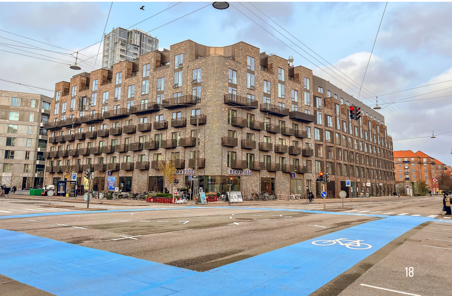
Figure 8: Affordable housing delivered through inclusionary zoning policies as part of the Bryggens Bastion project in Copenhagen
